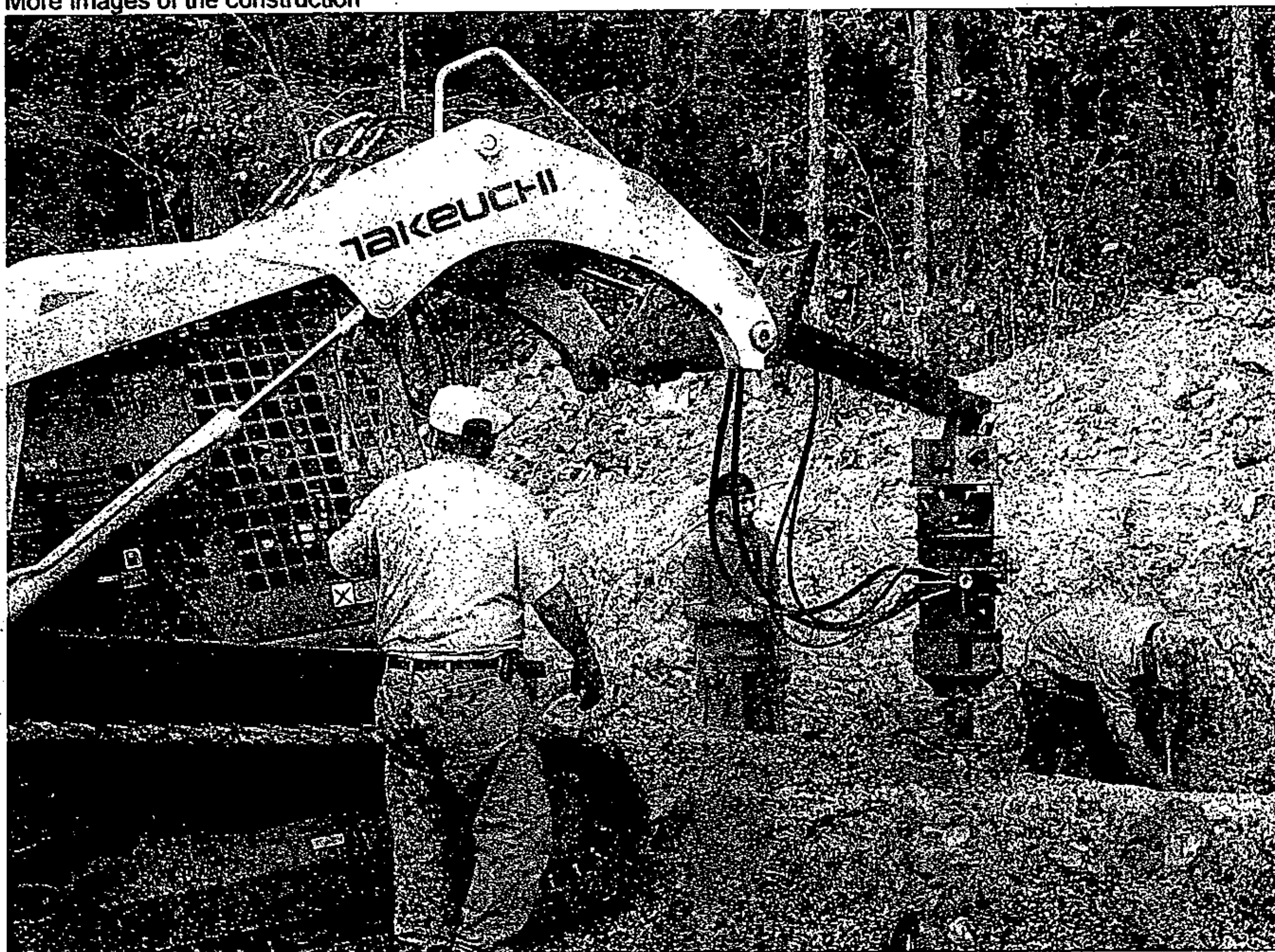
More images of the construction
