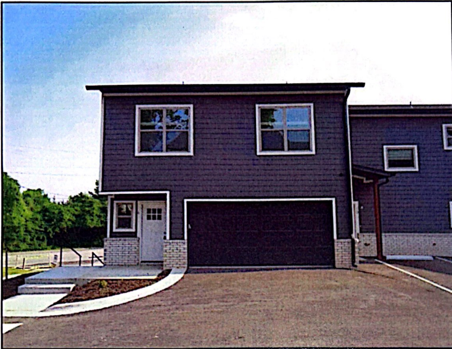
FRONT VIEW OF SUBJECT PROPERTY
