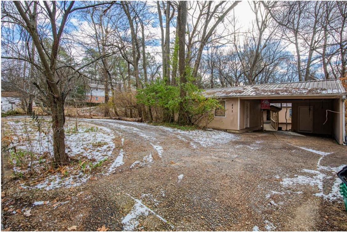
Carport & Storage Room - ALL Sides: Beige Siding, White Window/Door Trim, White Gutters, and Burgundy Roof
