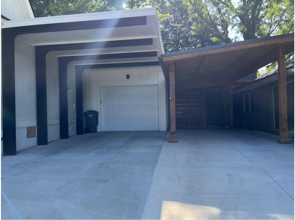
Figure 4: Applicant Photo, Downtown Example of Driveways on Property Lines
