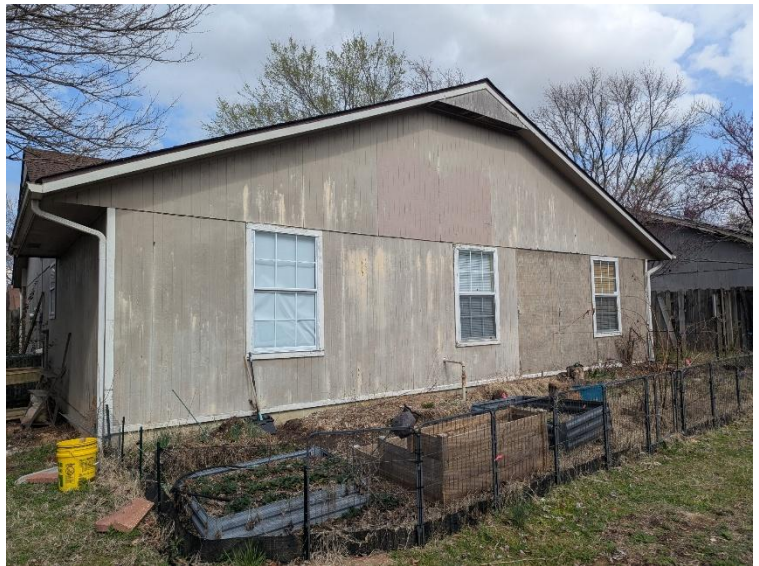
Rear of House (below/ South Facing)
