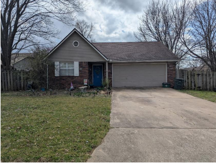
Front of House (facing North)
