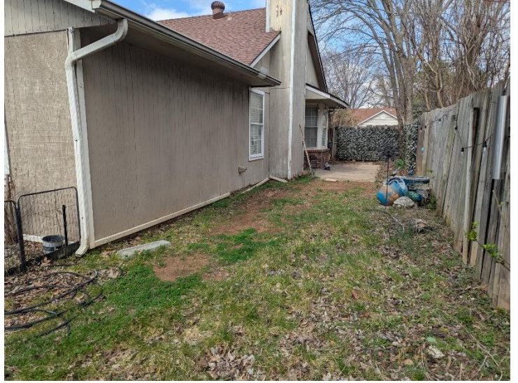
East Side of House (below)
