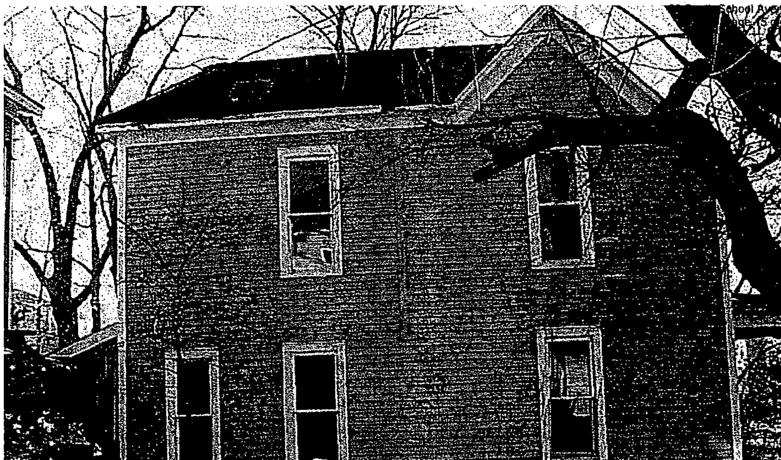
50 S. School Ave., 01-03-06, north elev. & roof
