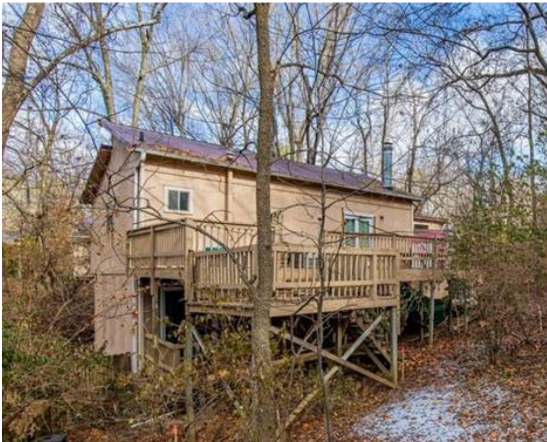
Back of House: Beige Siding, White Window/Door Trim, White Gutters, Burgundy Roof, and Tan Wood Decking
