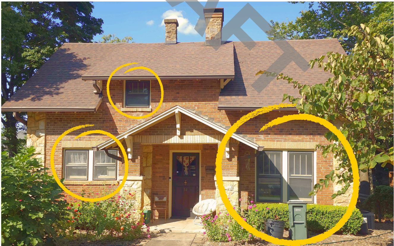
Figure 9. Example of existing windows on 14 Davidson
