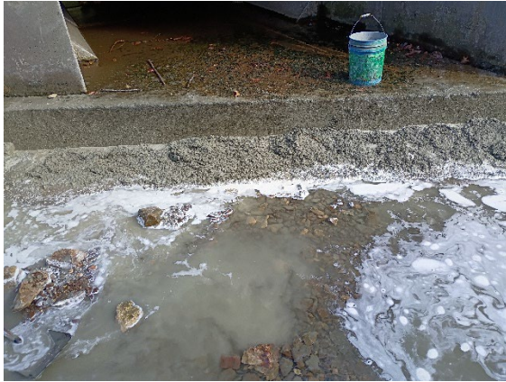
Picture 15:Box Culvert Foundation Repair
