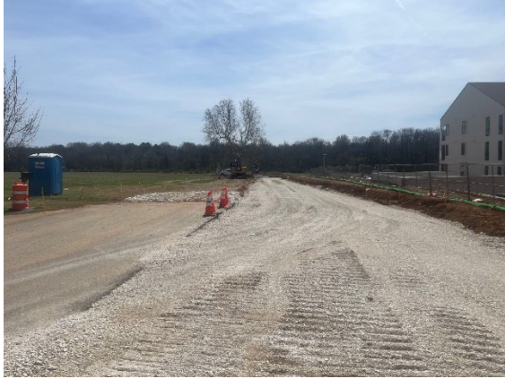
Picture 13: Hamstring Trail Construction Access
