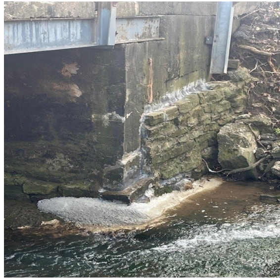
Picture 10: Bridge Foundation Repair
