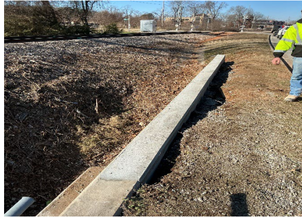
Picture 16:Retaining Wall Repair
