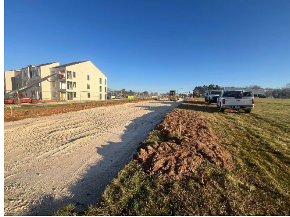
Picture 14: Hamstring Trail Construction Access
