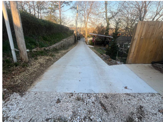
Picture 18:Completed Alley
