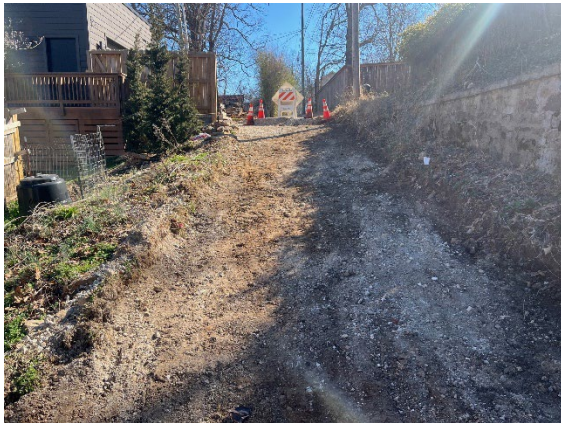
Picture 17:Alley Excavation
