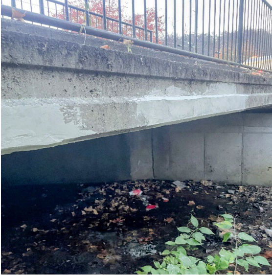
Picture 9: Concrete Bridge Patching
