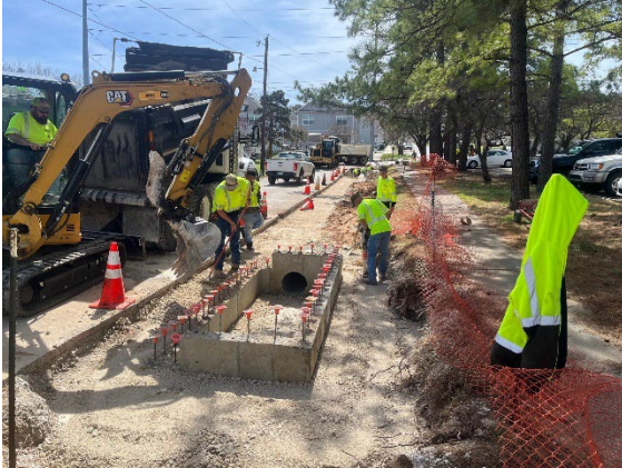
Picture 19: Cleveland St. Improvements
