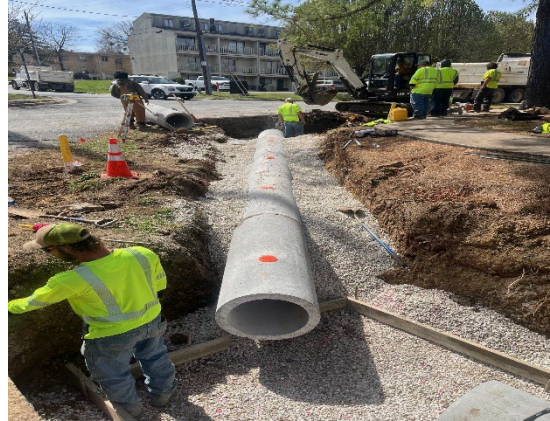
Picture 20: Cleveland St. Improvements
