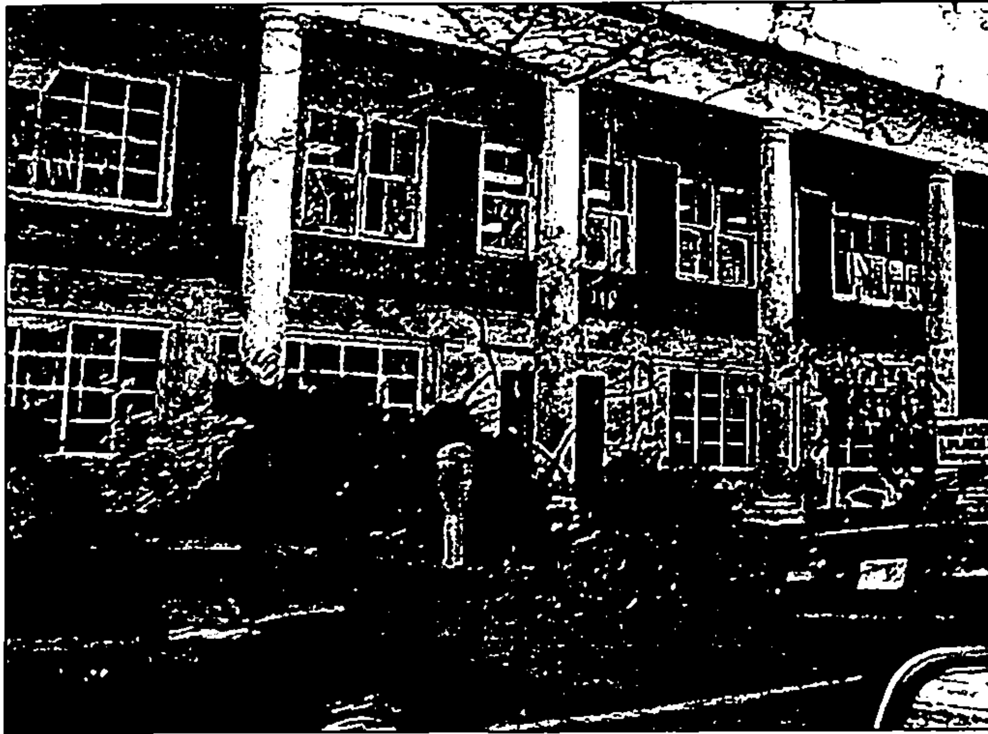
Existing structure facing East Ave.
