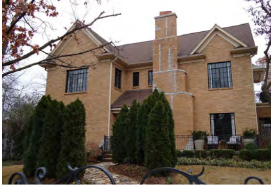
Figure 17. Hathcock House. The house is a contributing resource in the Washington-Willow NRHP Historic District.
