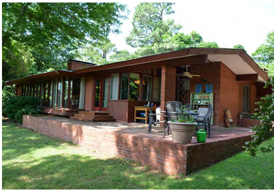
Figure 22. Heffelfinger-Freund House. The house was determined eligible for the ARHP in 2018. Source: AHPP. H
