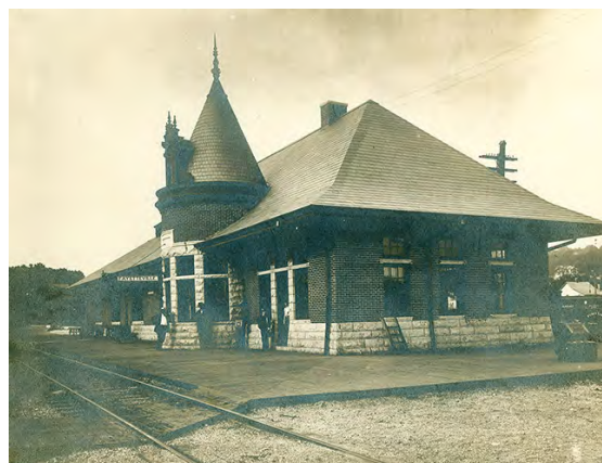
Figure 35. Fayetteville Frisco Depot. The Fayetteville Frisco Depot pictured ca. 1910. Source: Encyclopedia of Arkansas. N
