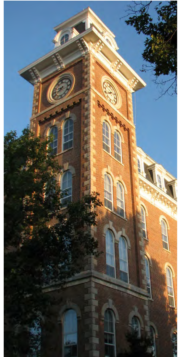
Figure 12. Old Main. One of the first buildings listed in the NRHP in 1970. Source: Brandon Rush E
