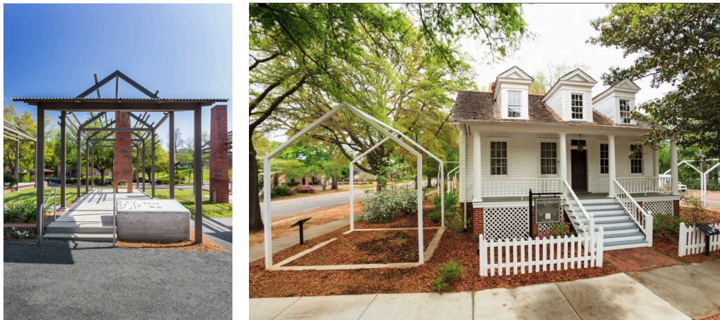
Left: Smokey Hollow commemoration in Tallahassee, Florida, depicting the building outlines of lost shotgun houses. Right: A “ghost structure” at the Mann-Simon Historic Site in Columbia, South Carolina; 5
