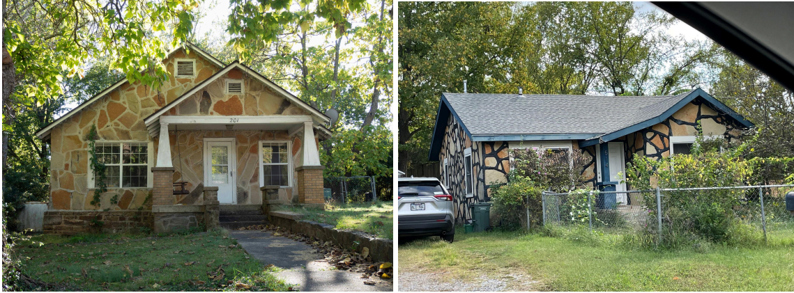
Left: 201 E. Huntsville Road, a Giraffe Rock bungalow (Resource 248). Right: 514 S. Willow, a Giraffe Rock house with blue/black mortar (Resource 371)
