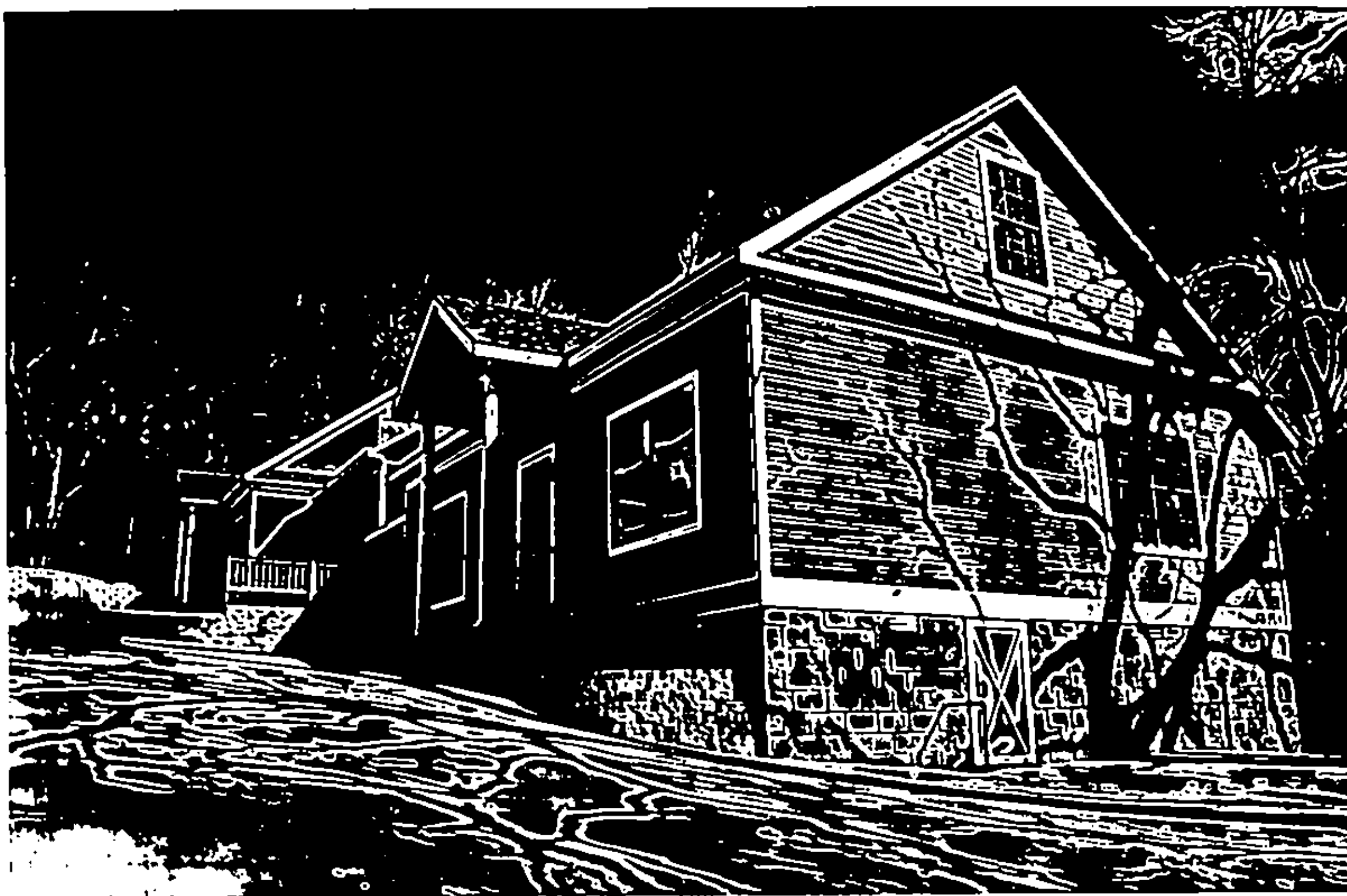
Olive Street Cottages -- $560,000
