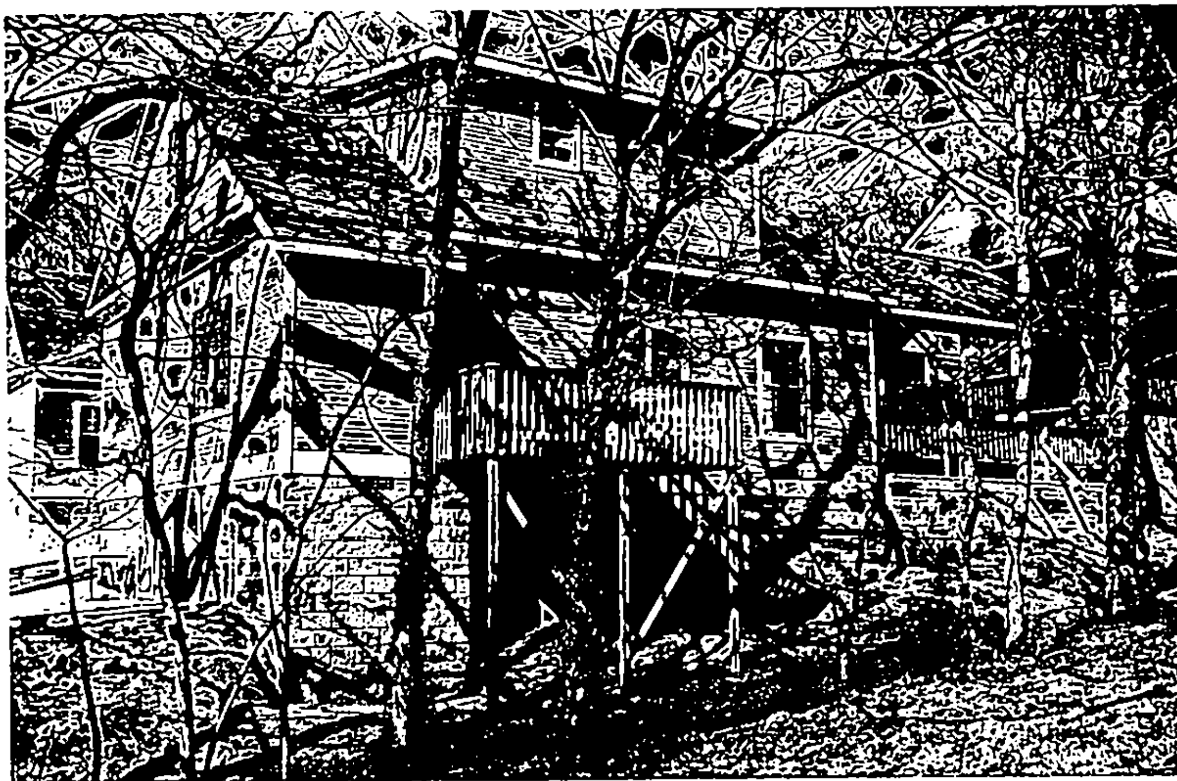
Olive Street Cottages – Rear Elevation
