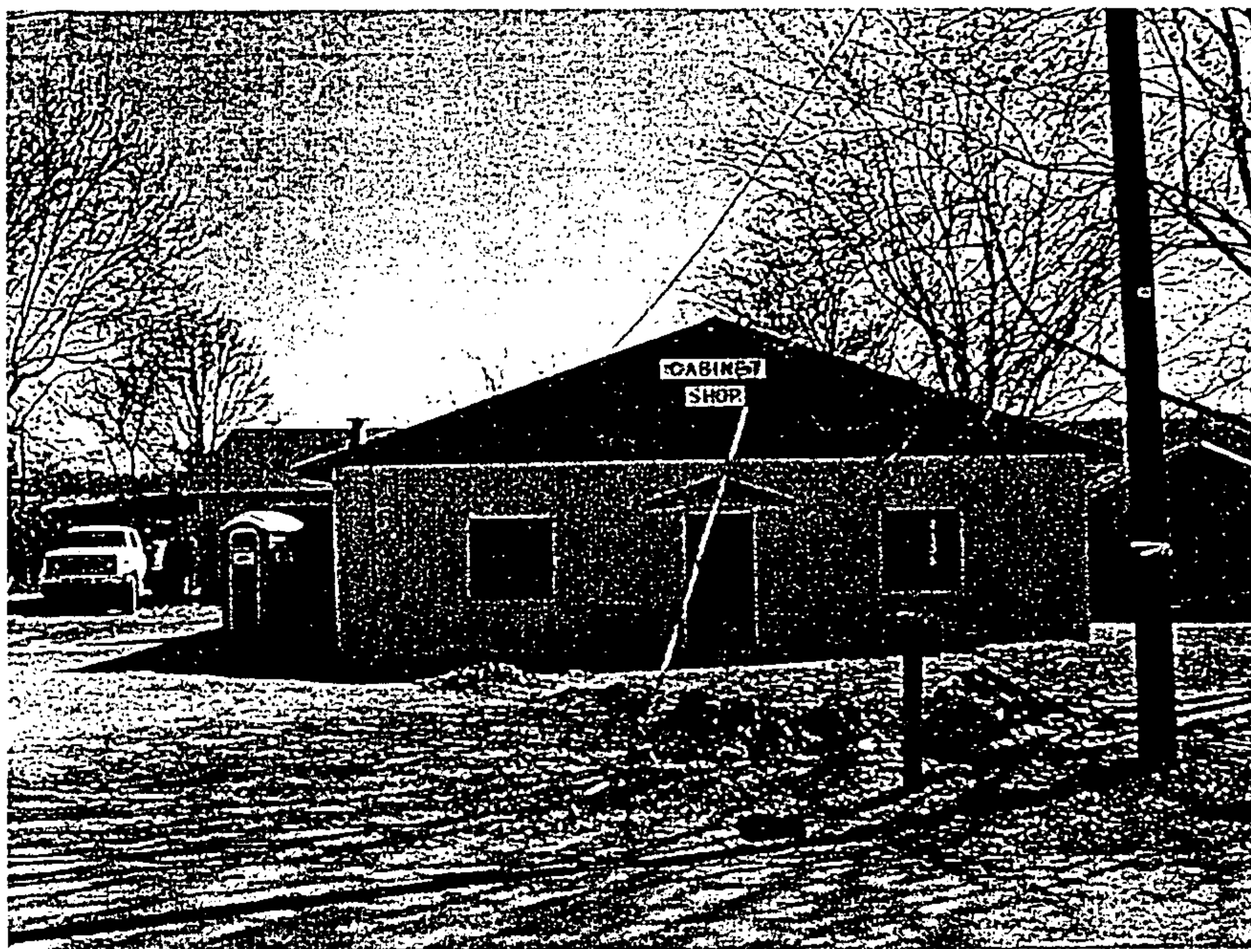
View of existing facility from Futrall Drive looking east
