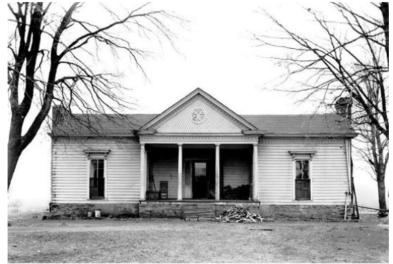
Figure 43. The ca. 1835 Waxhaws Hall (demolished) was built by second Governor of Arkansas, Archibald Yell. Source: University of Arkansas. s
