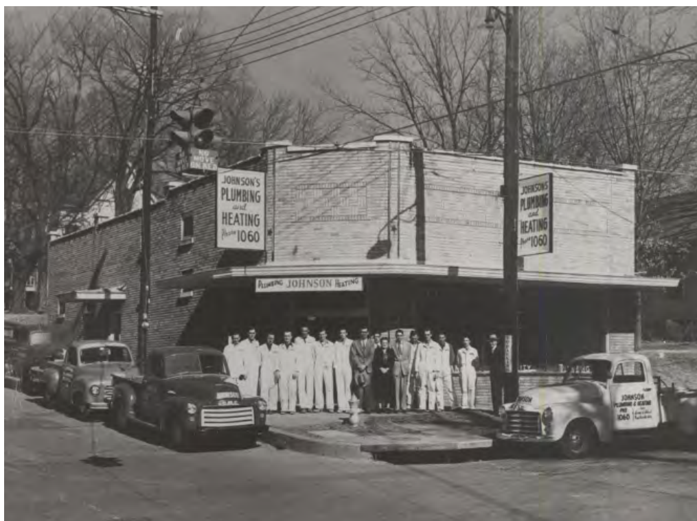
Figure 55. Johnson Plumbing. The Opening of Johnson Plumbing Presently known as the High Roller Cyclery located in the Meadow Spring NRHP Historic District.
