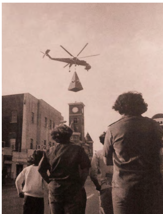
Figure 46. Steeple Replacement. Replacement of the Washington County Courthouse Steeple in 1974. Source: Washington County, Arkansas. v
