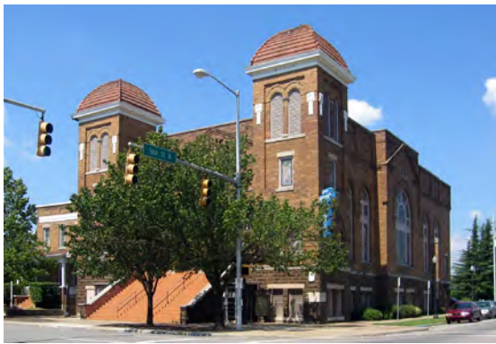
Figure 18. Sixteenth Street Baptist Church The church is one of numerous resources that contribute to the Civil Rights MPS in Birmingham, Alabama. Source: John Morse. 6
