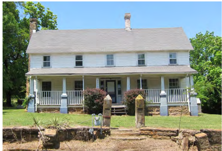
Figure 83. Thomas-Tharp House (1854). This house was placed on the Arkansas's Most Endangered Places list in 2018.
