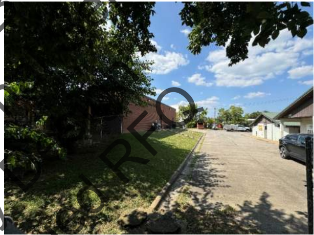
Back of existing shelter
