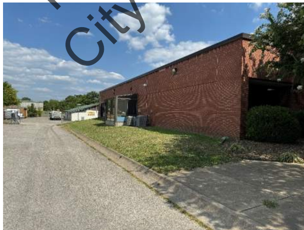
Side of existing shelter
