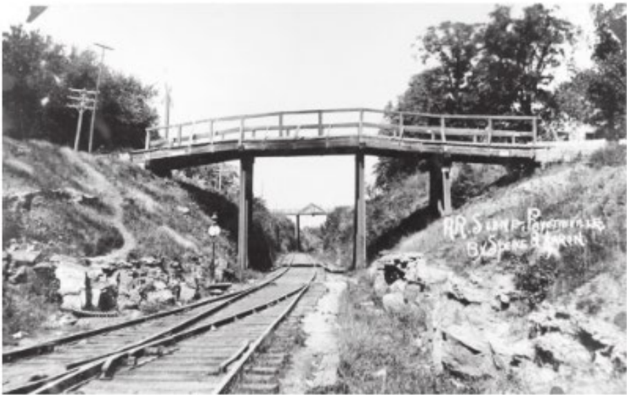
The Frisco Cut, with an early wooden Lafayette Street bridge in the foreground and the Maple Street bridge in the background, in about 1909. The two bridges were replaced with concrete bridges that are now in the National Register of Historic Places. Photo by Speece & Aaron. Courtesy Shiloh Museum of Ozark History, Mrs. Kenneth Tillotson Collection, S-90-91-1.
