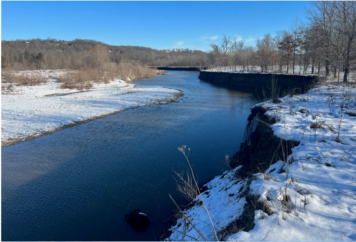
Highly degraded channel pre-construction and restored channel post construction.
