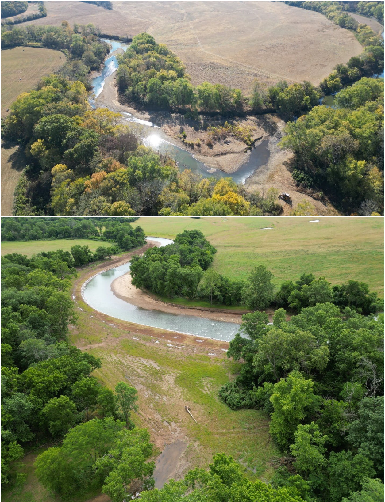
Pre and Post Construction photos showing the old lake bed before construction and the newly constructed channel post construction.
