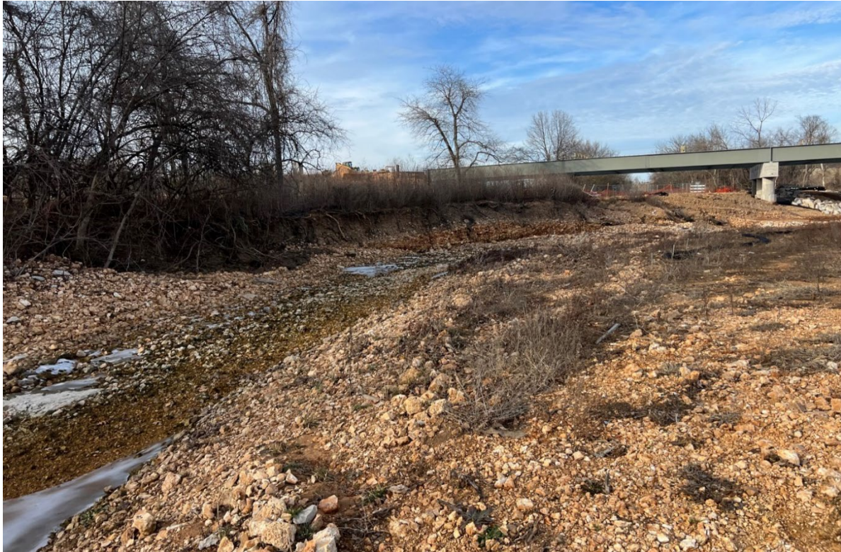
Photos just upstream of the newly constructed bridge showing the degraded channel and restored channel.
