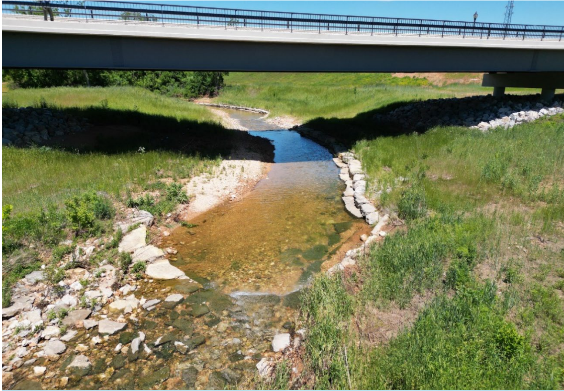
Post Construction Photos showing the stream restoration work both upstream and downstream of the newly constructed bridge.
