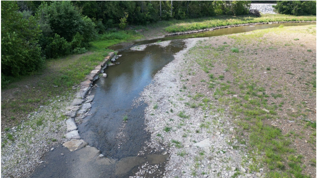
Restored Channel with J-hook grade control structure and toewood bank protection.
