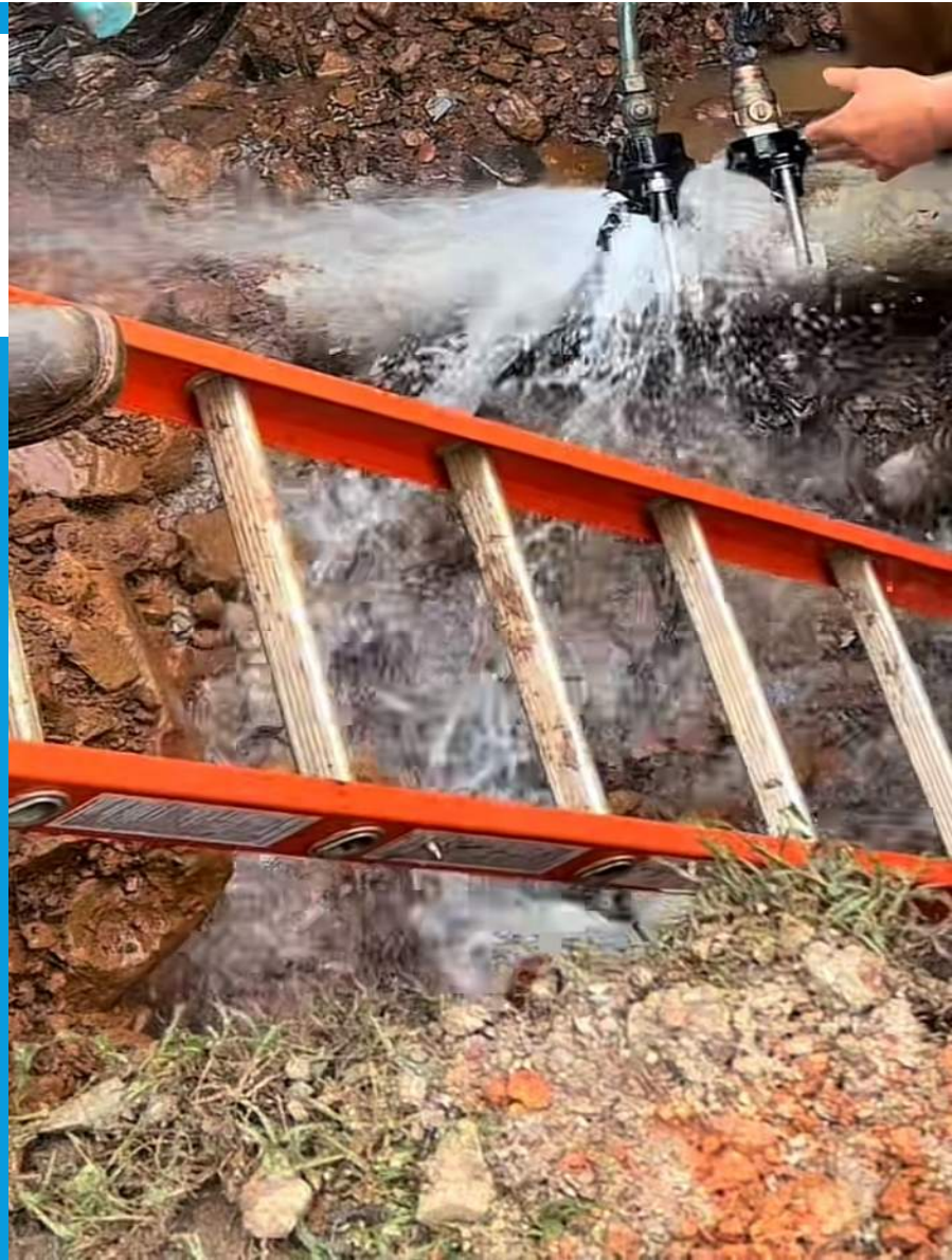
2" main repair utilizing hydro excavation (left) and a leaking service saddle being replaced (right).
