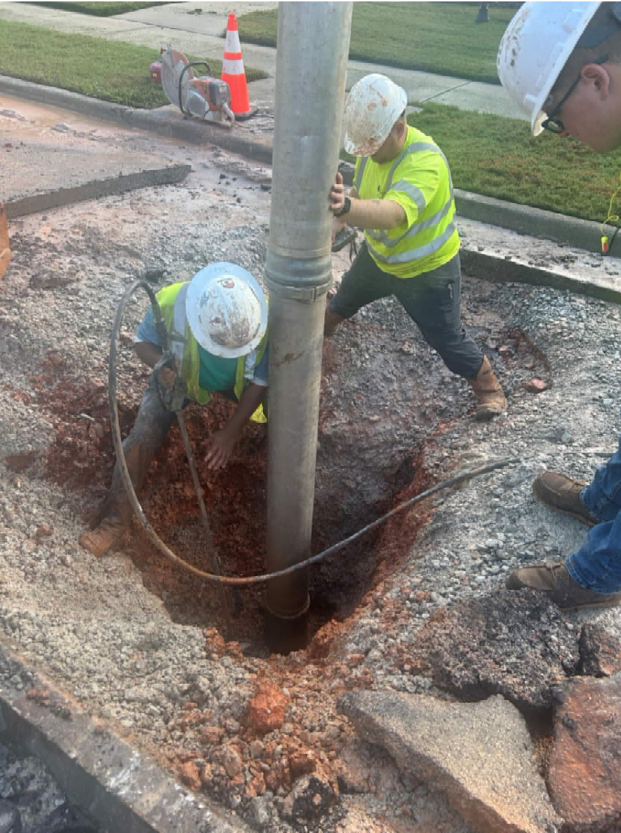
2" main repair utilizing hydro excavation (left) and a leaking service saddle being replaced (right).
