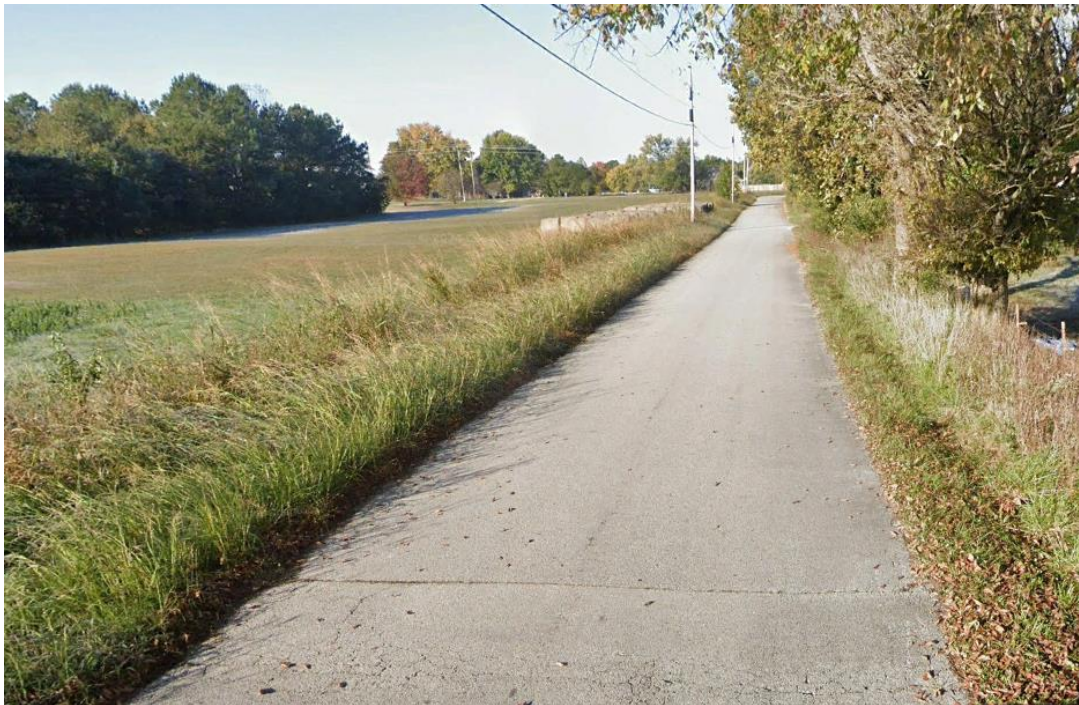
Photo of Dot Tipton Rd, near the western new proposed access.
