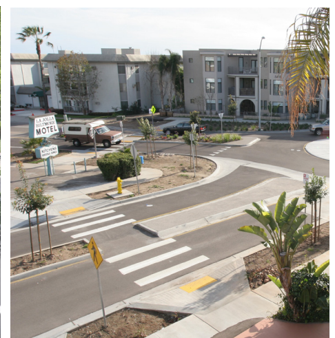
Median and pedestrian refuge island near a roundabout. Source: www.pedbikeimages.org / Dan Burden
