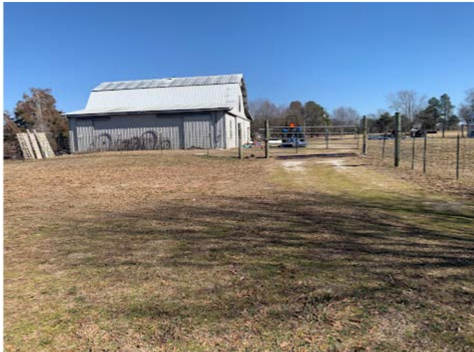
SUBJECT PROPERTY – LOOKING EASTERLY
