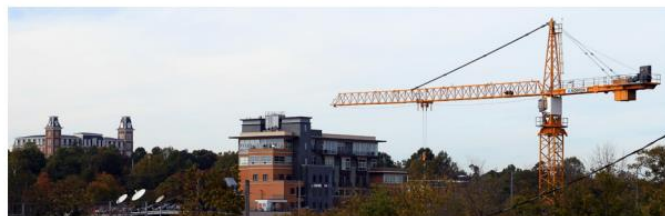
Photo 3.8 - Construction in Downtown Fayetteville
