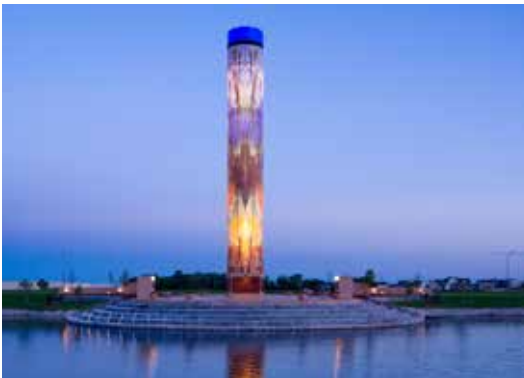
Free-Standing Installation. Paragon Prairie Tower, Des Moines*
