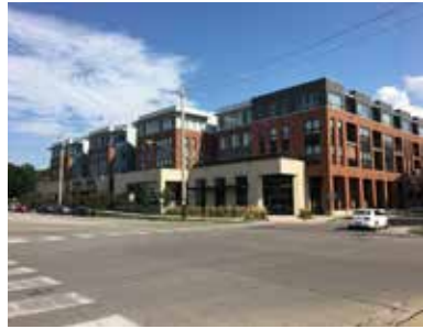
Screening parking with projecting storefronts. This concept on a significant street permits both at-grade parking and street-facing retail. (Iowa City, IA)
