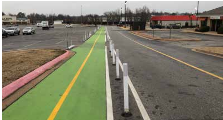
Pilot cycle track in Fiesta Square parking lot. A pedestrian and bicycle link along a new Plainview-Appleby connector is a critical part of the transportation network.
