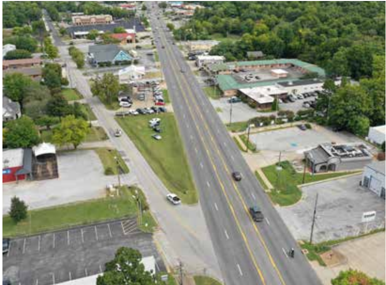
Divergence of Green Acres and North College. Redesign of this intersection to provide a 90 degree angle will both improve safety and create an open space “triangle,” a central commons that can serve neighboring residential development.
