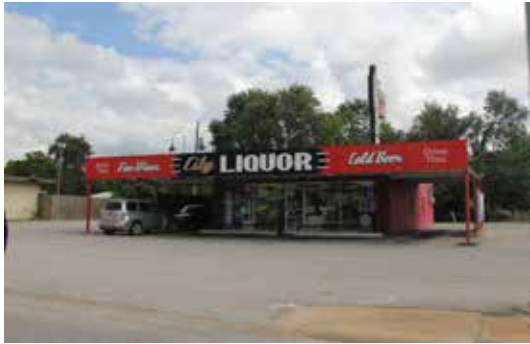
Commercial preservation. City Liquor, Fayetteville
