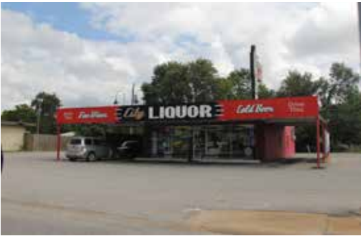
Commercial preservation. City Liquor, Fayetteville
