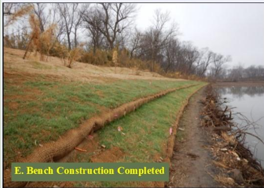
C. Toe Wood Bench Completed
