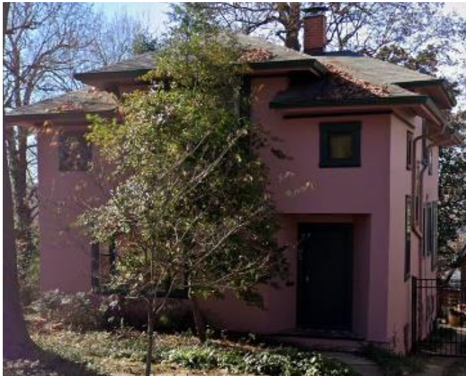
Prairie-inspired stucco dwelling with hipped through-cornice dormers, constructed ca. 1926 according to Washington County Assessor records. Appears in 1926 aerial image.
