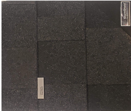
ARCHITECTURAL SHINGLE ROOF
