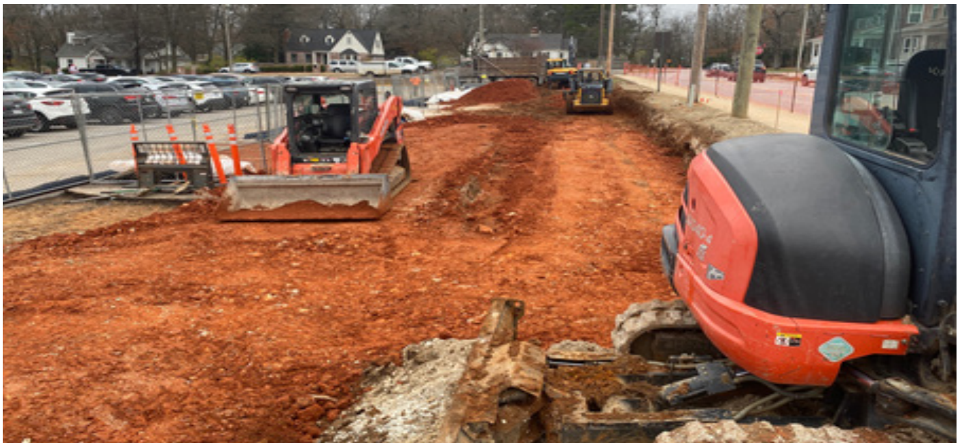
Excavation at retaining wall preparing for new curb, gutter, and the Iconic U of A Senior Sidewalk.
