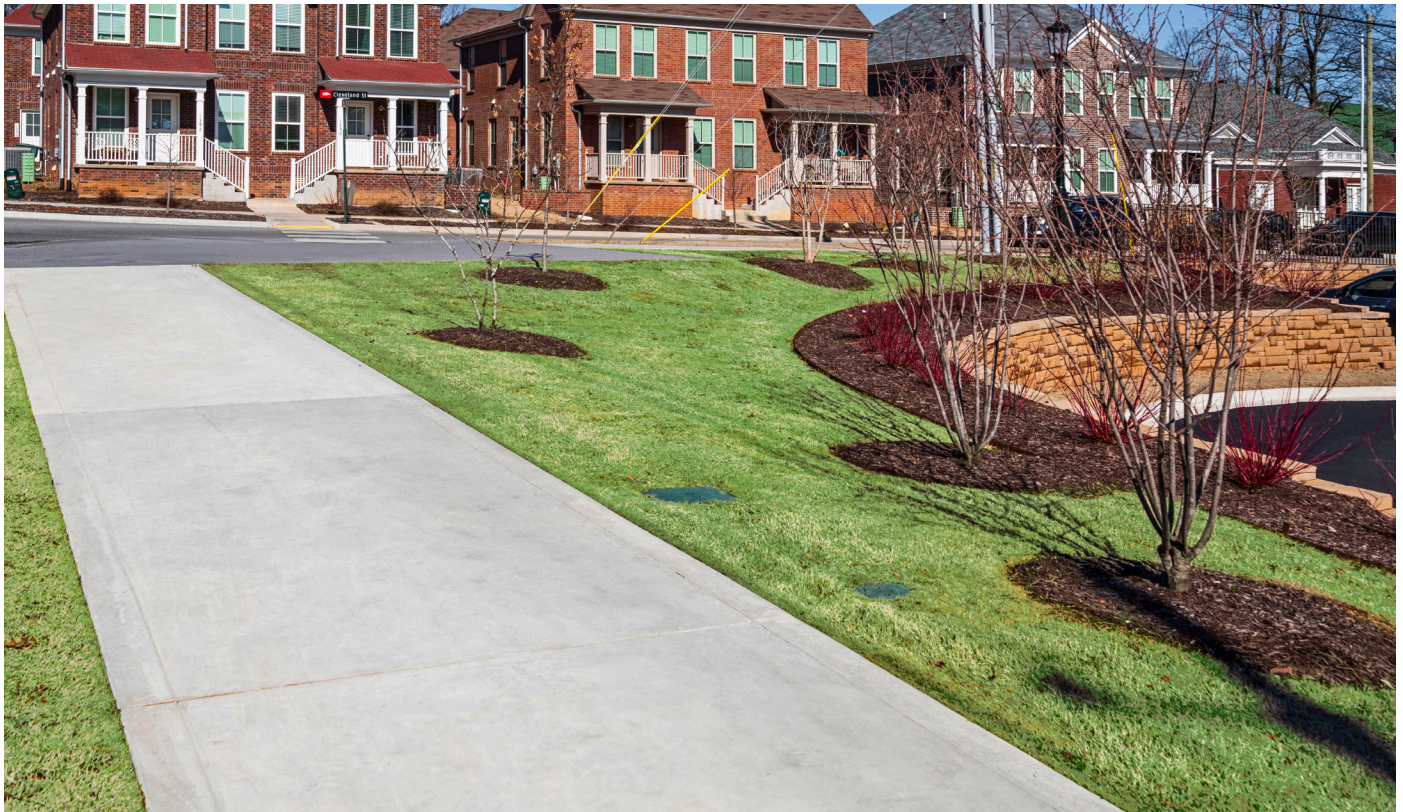
Landscaping, senior sidewalk and retaining wall that were all a part of this 2020 – 2025 Senior Sidewalk Project just south of a residential area off Razorback and Cleveland Streets.
