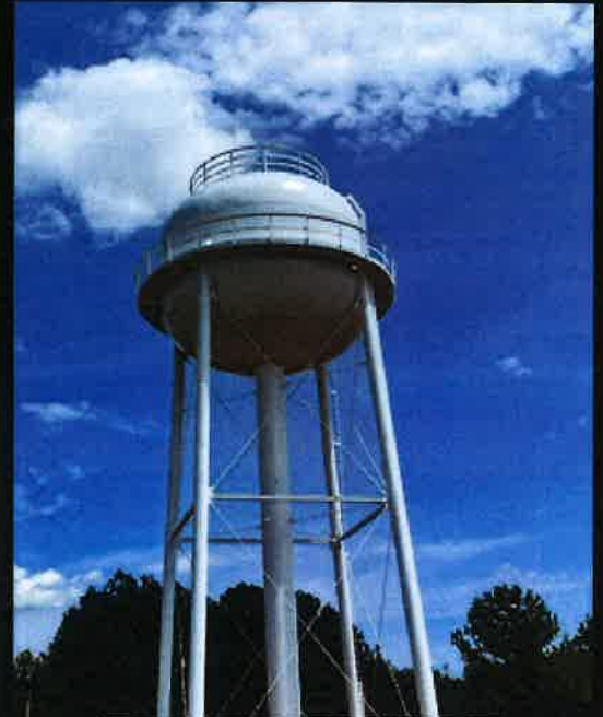
New Benson Water Tank 100,000-gallons Completed in 2023 for $1,155,000
