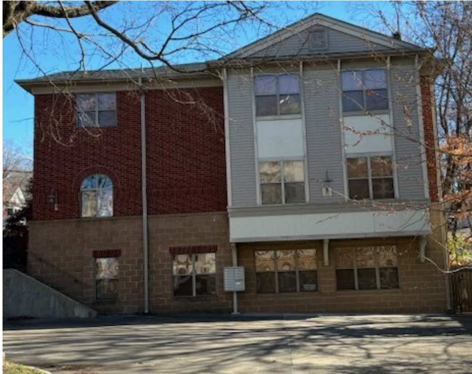
Lafayette Condo Building – 6 units - 3-stories
