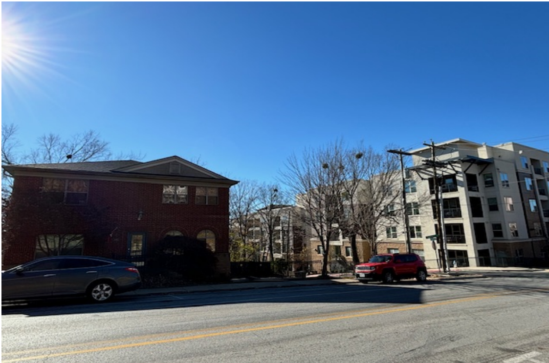
Lafayette street view (Lafayette Condo Building & YOUNion Apartments)
