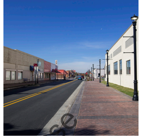
Emma Avenue - $1M Springdale, AR
