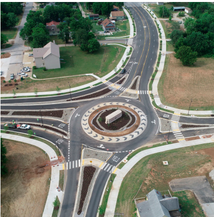
Monte Ne Road Realignment - $9M Rogers, AR
