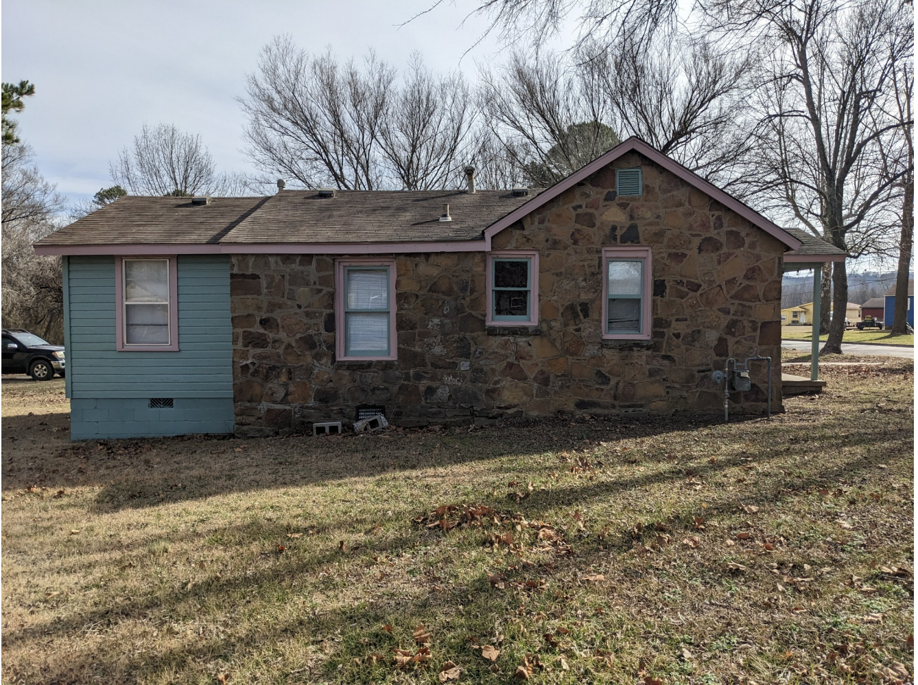
Side View (From Northwest)
