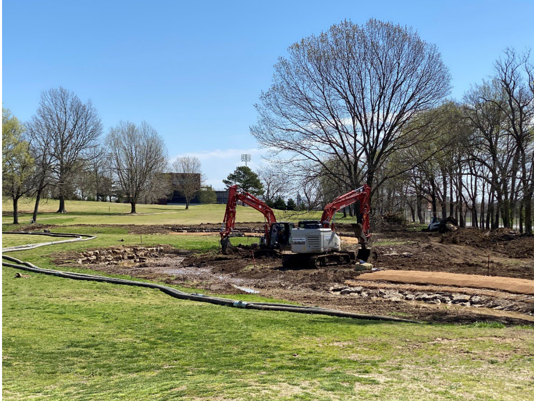
Photo 3. Sager Creek stone toe protection during construction. NSS employed a pump-around technique during construction to preserve water quality and manage water onsite.
