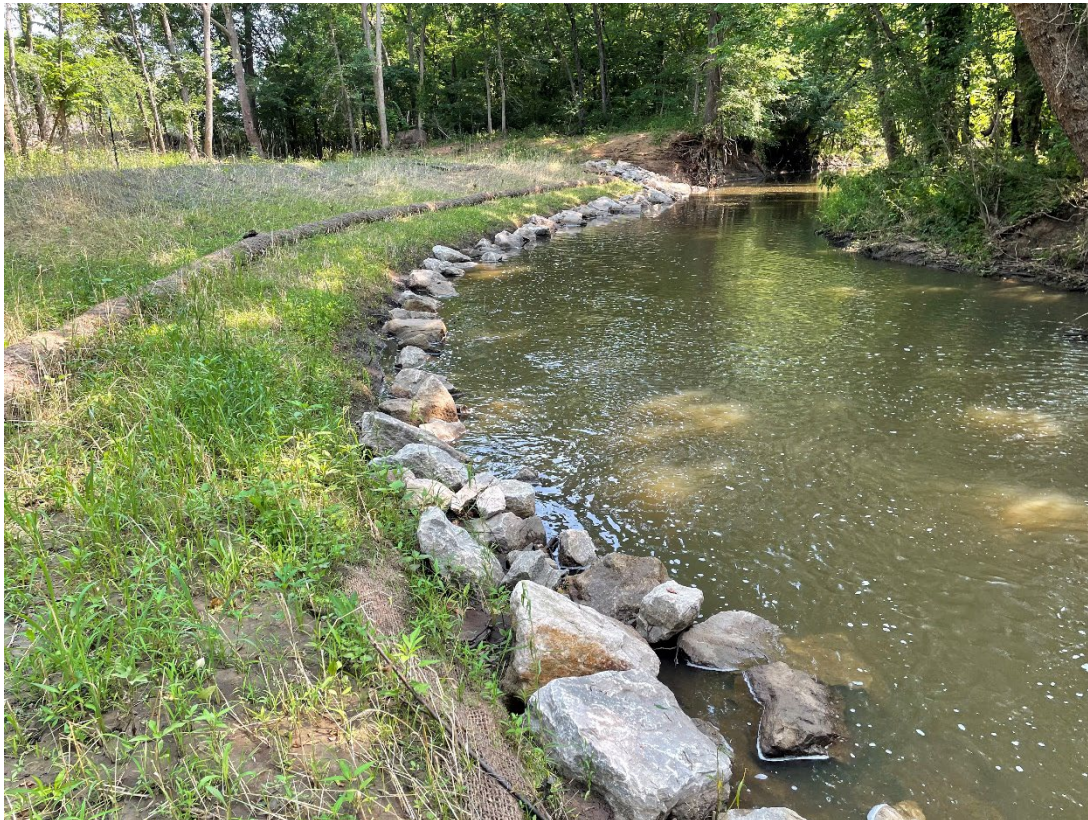
Photo 5. Cloud Creek stone toe protection after first major flood, several months post-construction.
