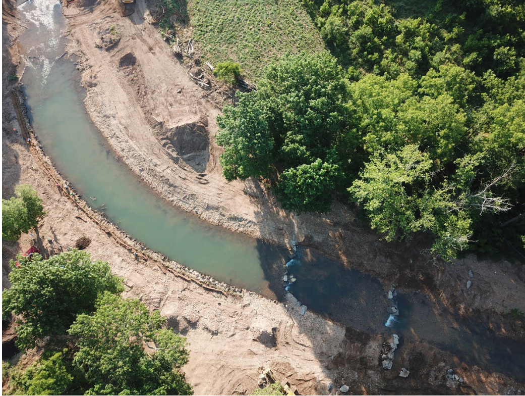
Photo 1. Osage Creek during construction. Overhead view shows multiple stone vanes and wood toe protection shortly after installation.
