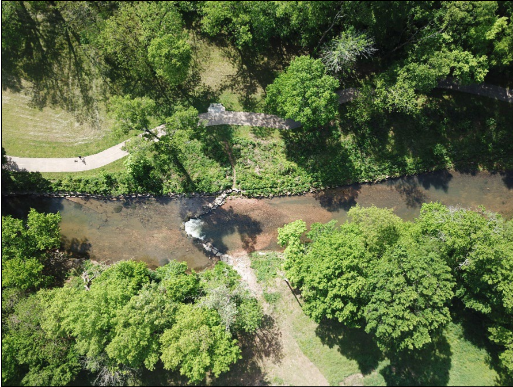
Photo 4. Osage Creek Cross vane 3 years post construction
