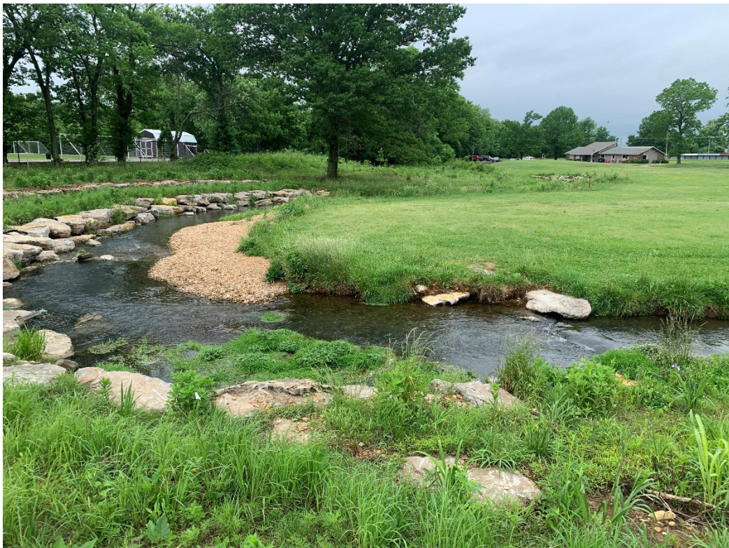
Photo 4. Sager Creek stone toe protection and j-hook structure with step-pools 1 year post construction.
