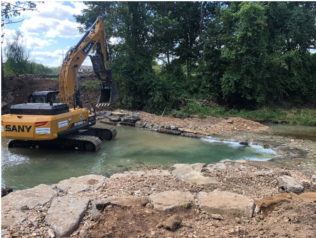
Photo 2. Osage Creek cross vane during construction.
