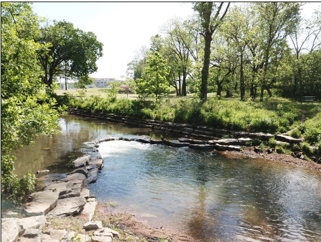
Photo 5. Osage Creek Cross vane 3 years post construction
