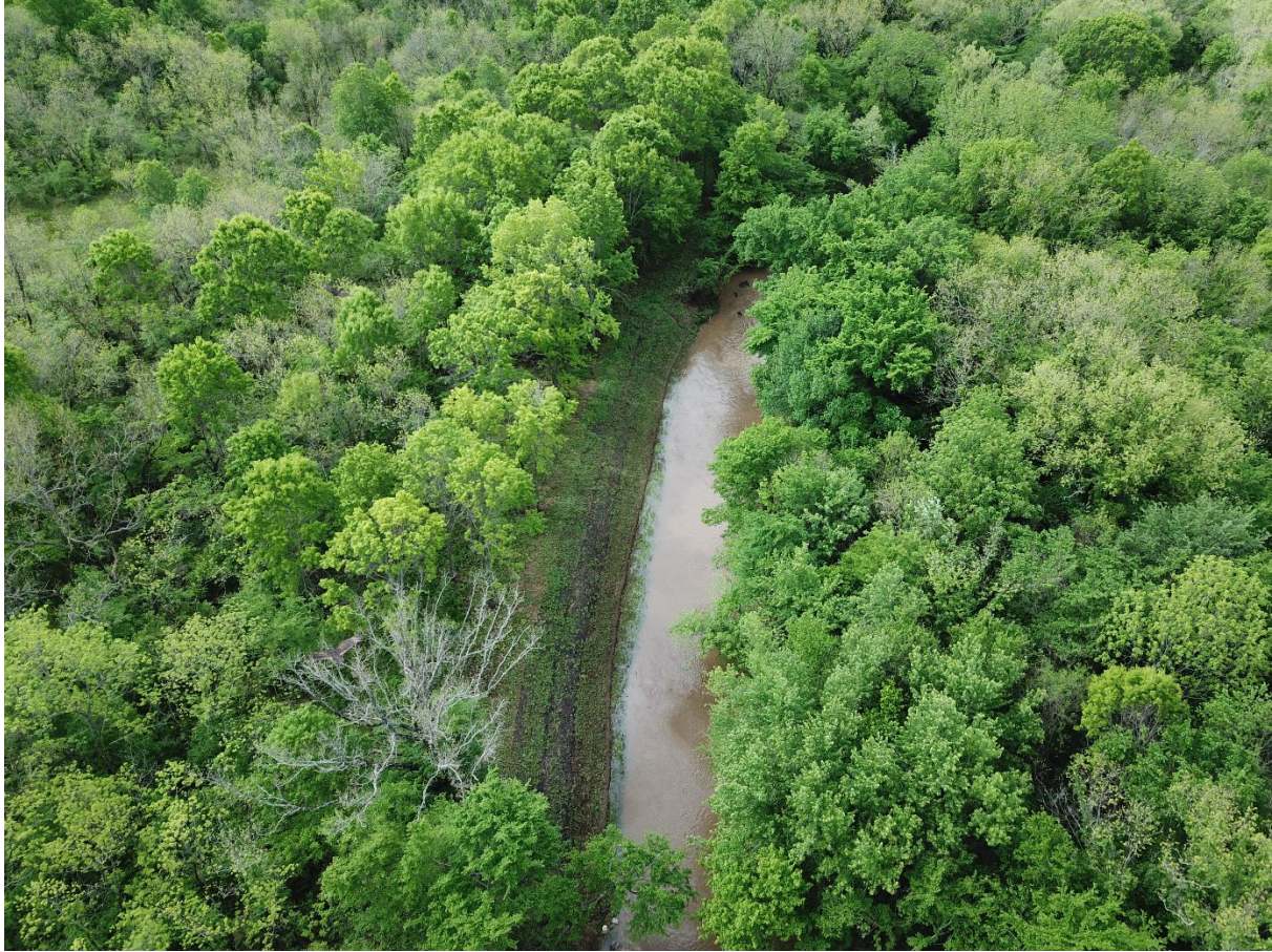
Photo 6. Above view of Cloud Creek stone toe protection after first major flood, several months post-construction.
