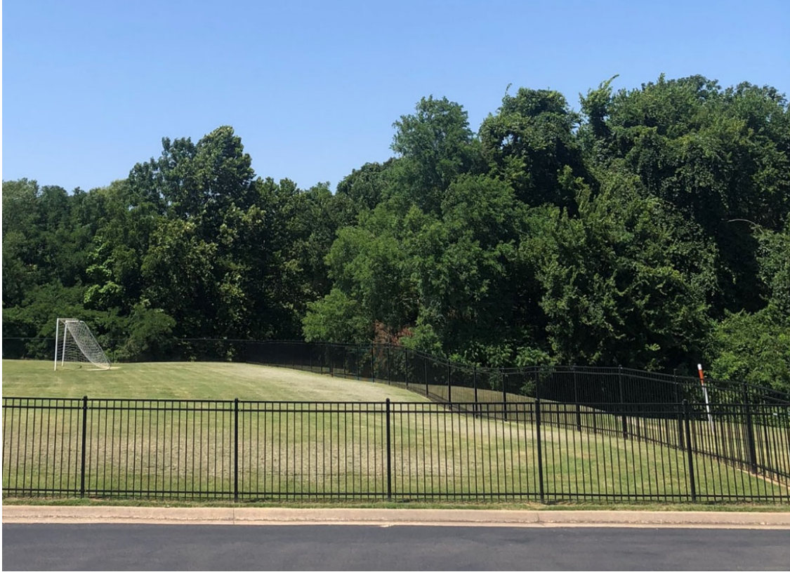
Existing fence at proposed location.
